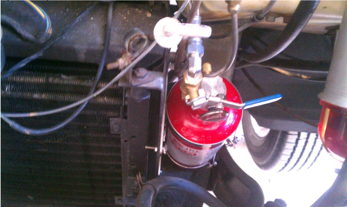
Cylinder in place
