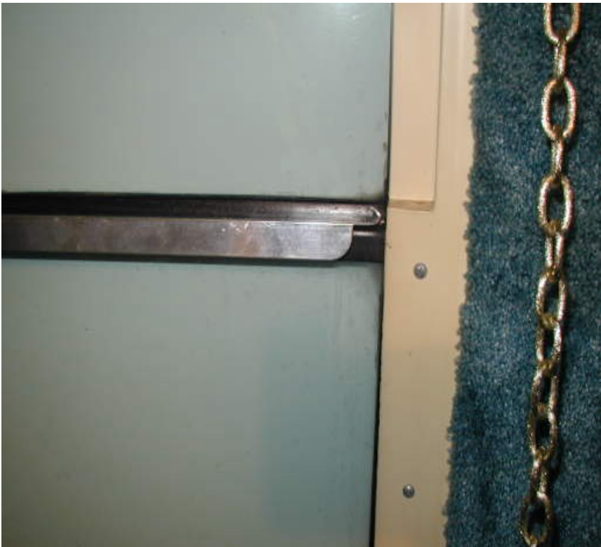
Picture 4: Place the top screen rail such that the end with the bend goes into the window frame tunnel.
